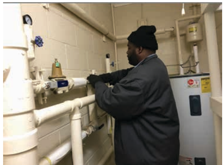
Draining water pipes at Milam Park.
