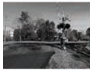
2. EXISTING FROM CHURCH STREET AT RAILROAD CROSSING
