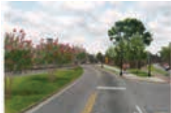
1. VIEW FROM CHURCH TO PONCE
