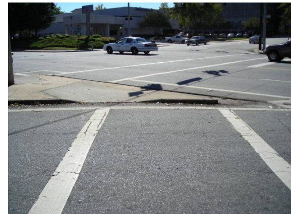
The walkability and bikeability assessments evaluated intersections and crosswalks
