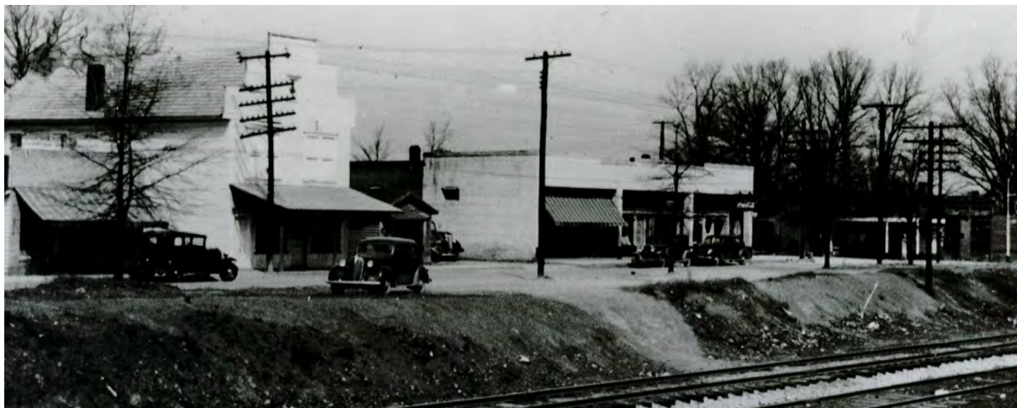
The Georgia Railroad running through Clarkston, Source: City of Clarkston
