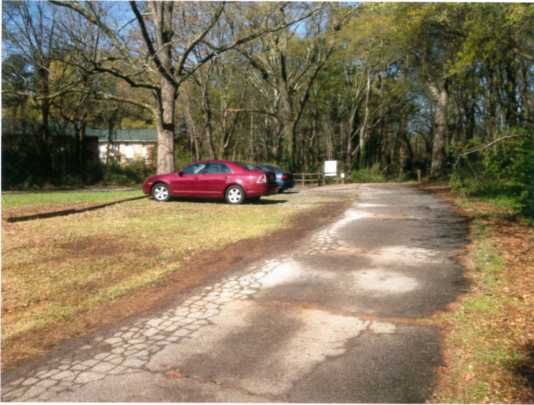
View of the unpaved parking area near the entrance from E. Ponce De Leon Avenue.
