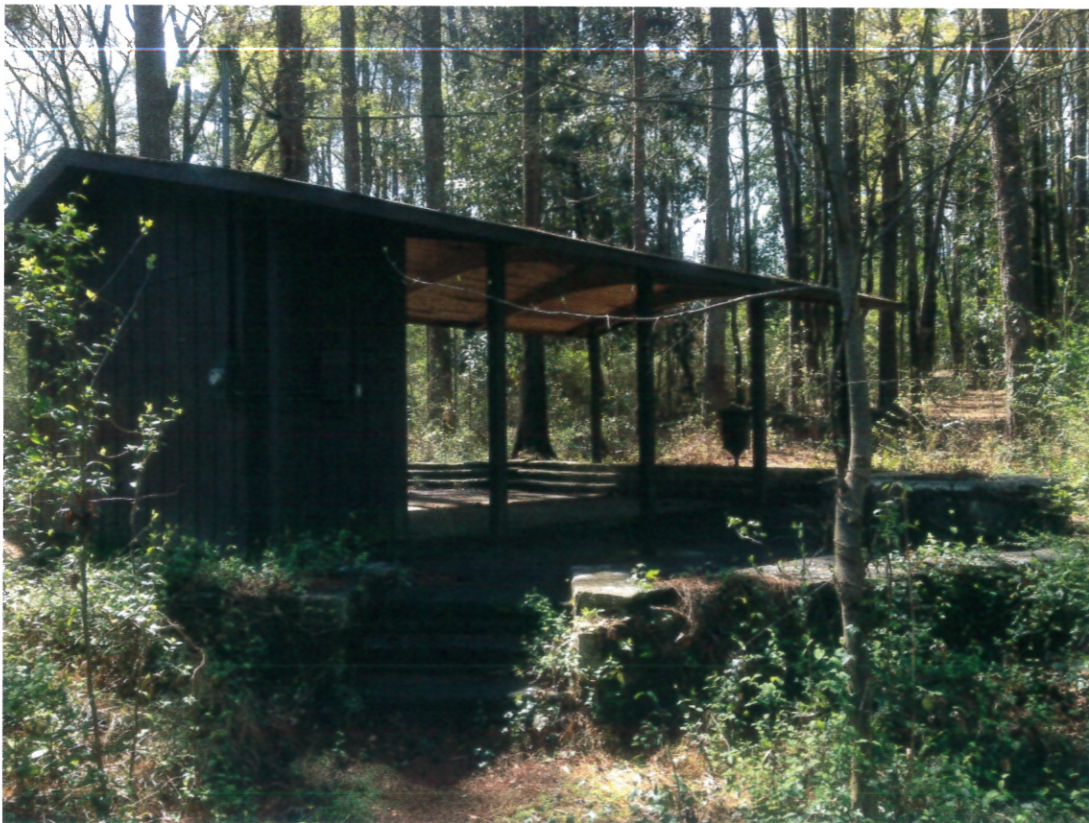
View of the existing picnic pavilion, restroom, fire pit and stone patio.
