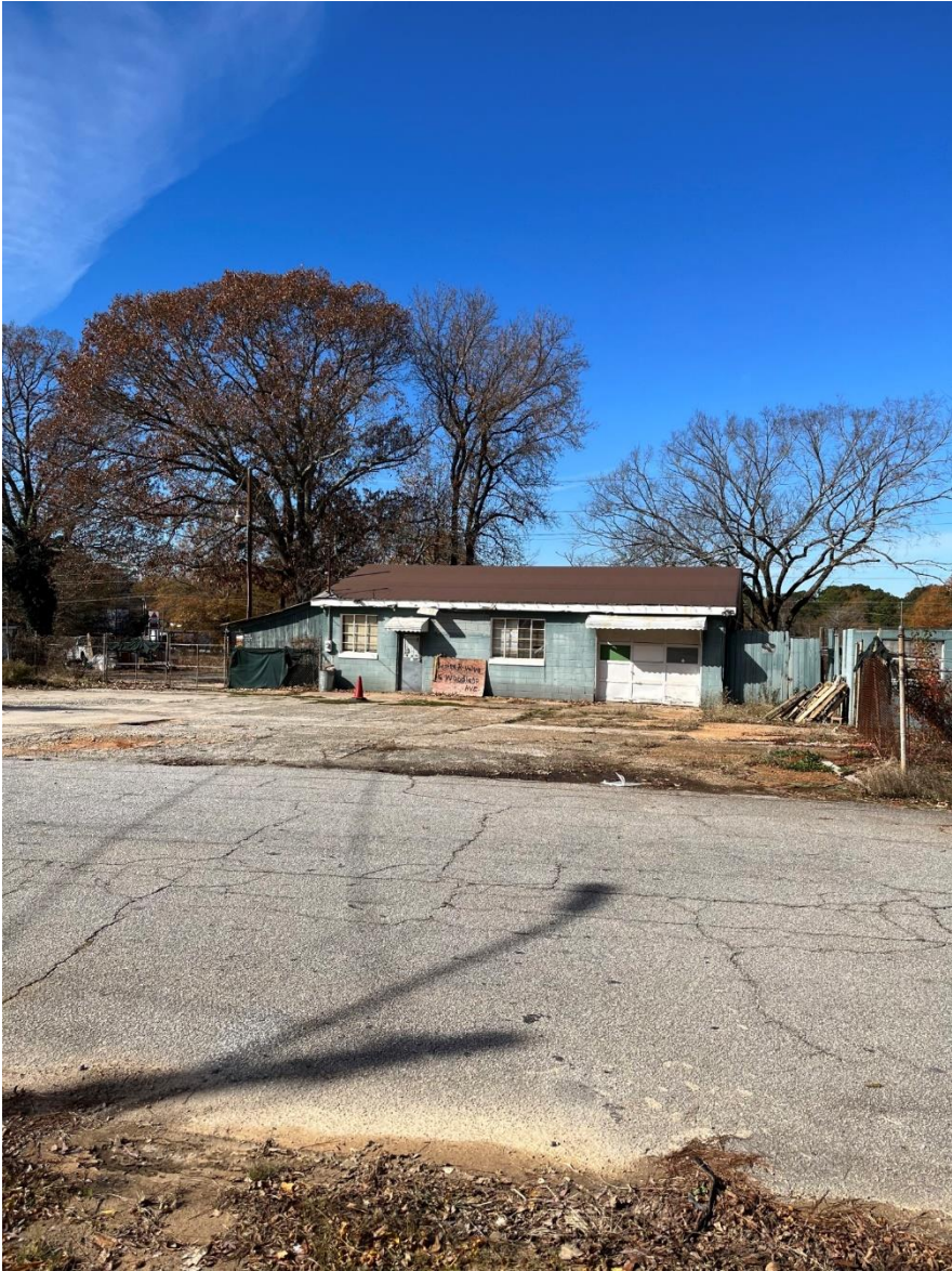
616 Woodland Avenue Scottdale, GA 30079 – Structure 2 of 2
