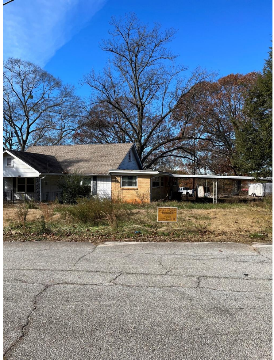
616 Woodland Avenue Scottdale, GA 30079 – Structure 1 of 2
