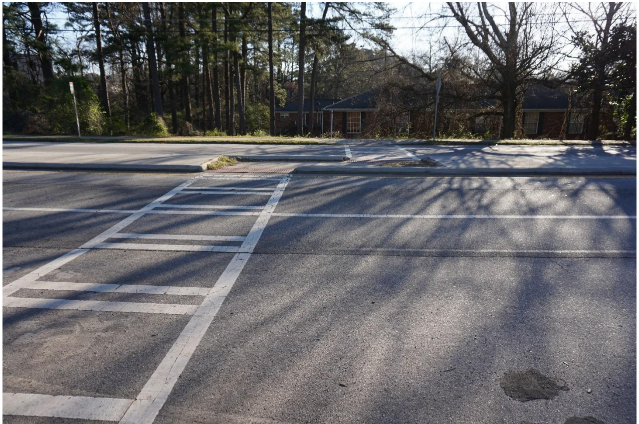
Vehicles were observed to travel at high rates of speed throughout the corridor along N. Indian Creek Drive. Pedestrian median refuges (above) have been added at key intersections. Additional signage and lighting and potentially a Rectangular Rapid Flashing Beacon Assembly or Pedestrian Hybrid Beacon are recommended to improve visibility of crossing pedestrians.
