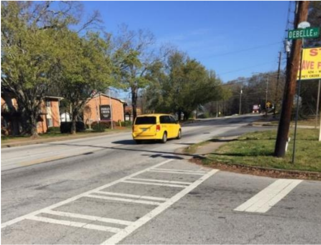
Crossings at Debelle street could be improved by re-stripping the crosswalks and adding detectable warning surfaces
