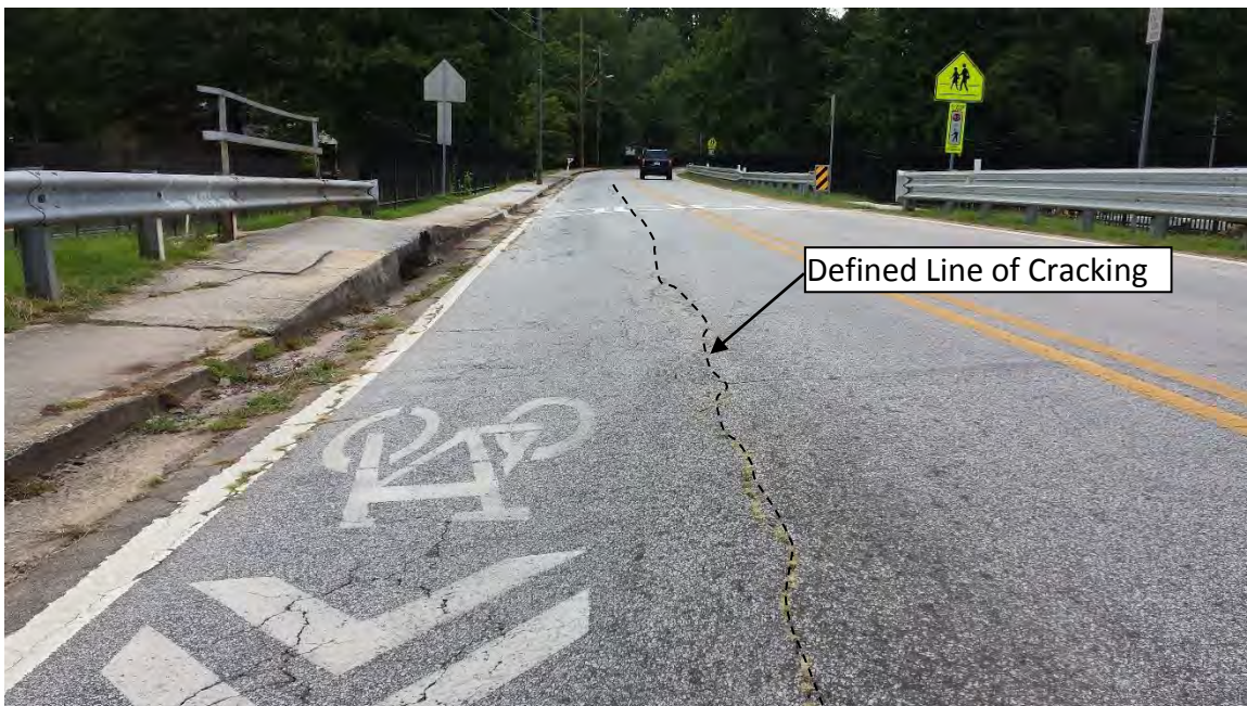
Norman Road – Facing West: Settlement and Cracking
