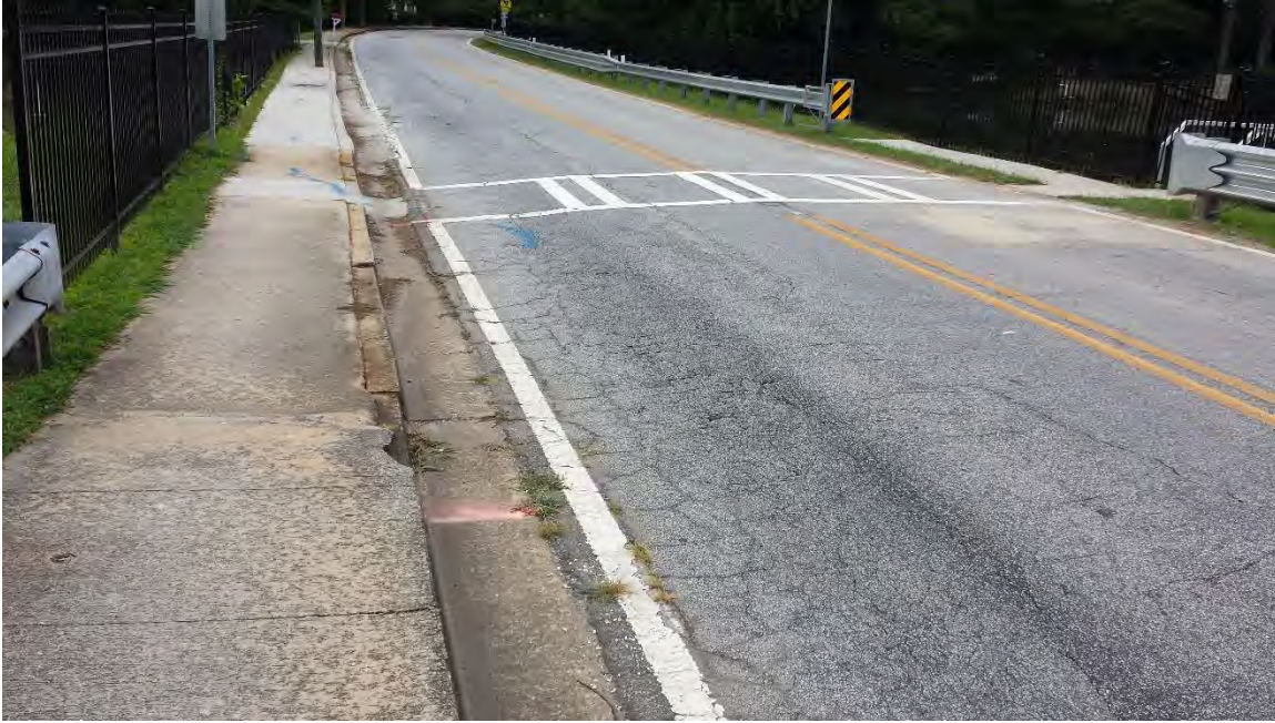
Norman Road – Facing West: Settlement and Cracking
