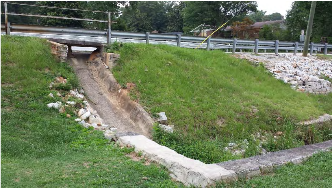
Emergency Spillway Flume; Facing Northeast
