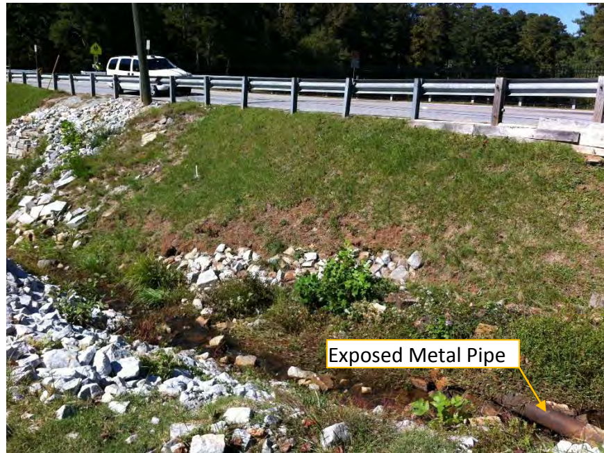
Sloughing of Downstream Slope; Facing Northwest
