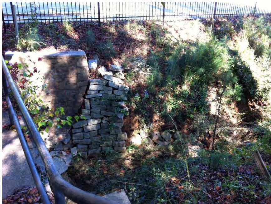
Damaged Retaining Wall, Steep Slope, and Sloughing at West End of Dam; Facing North
