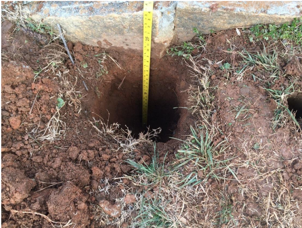
Side view of Test Pit #2
