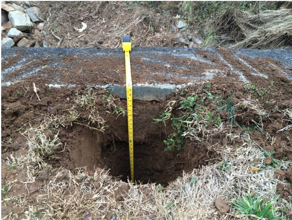
Side view of Test Pit #1
