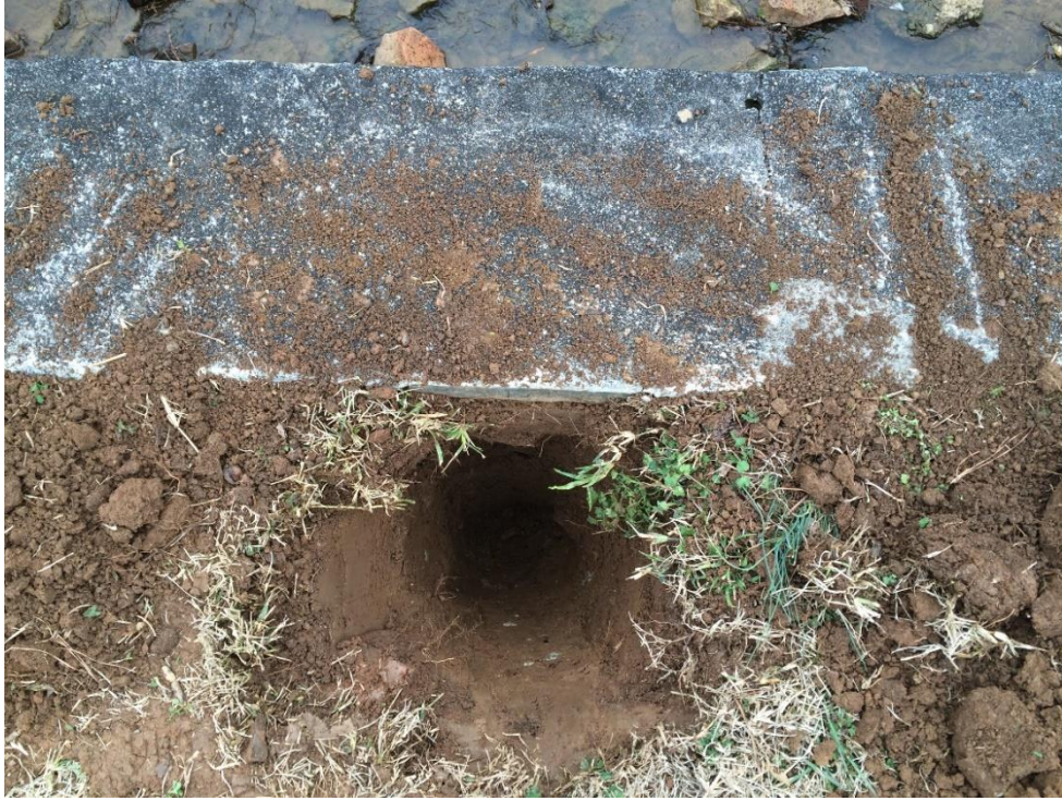
Top view of Test Pit #1
